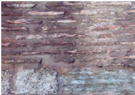
Crushed brick-lime mortar in Hagia Sophia
